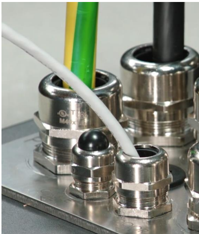
Figure 53: Tighten cable glands
