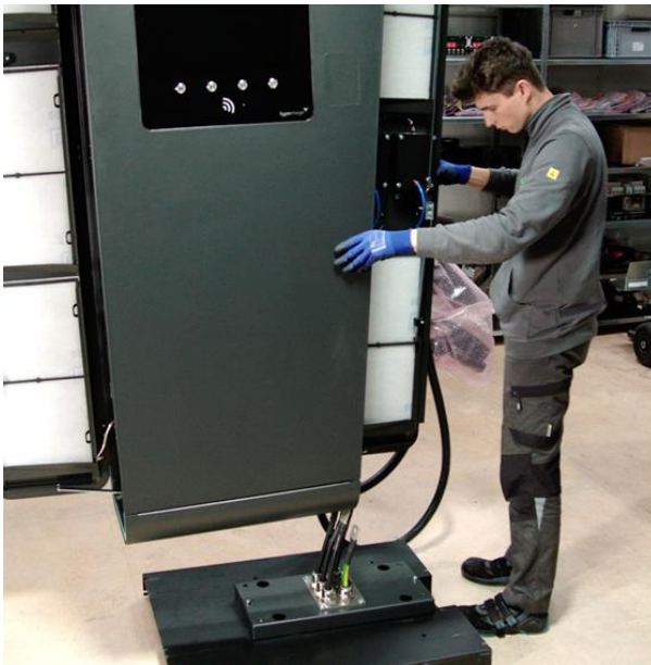
Figure 54: Positioning and attaching the HYC200 on the base
